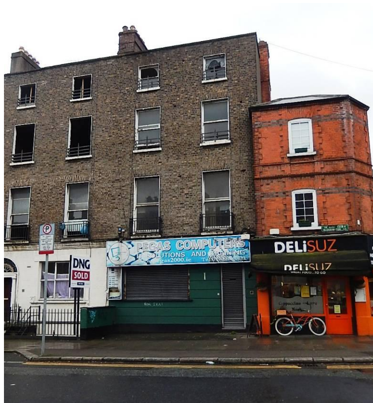
Photo of Structure
