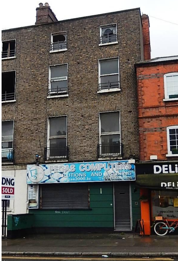
View of front façade to 58 Blessington Street
