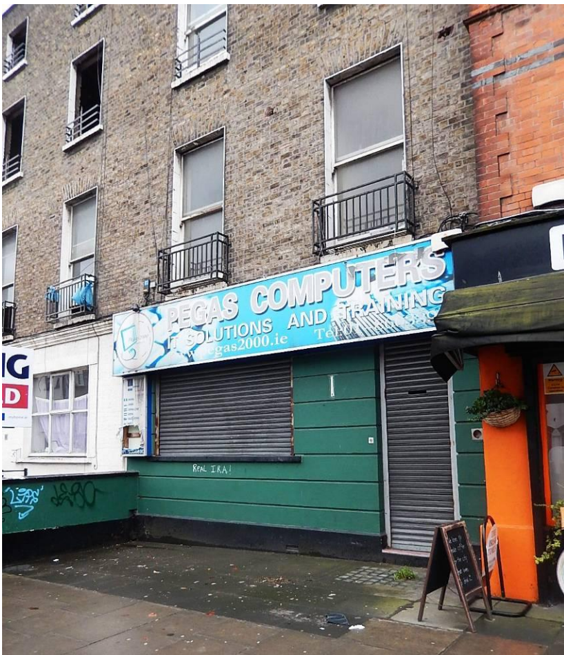
View of ground floor with later shopfront and upper floor windows.
