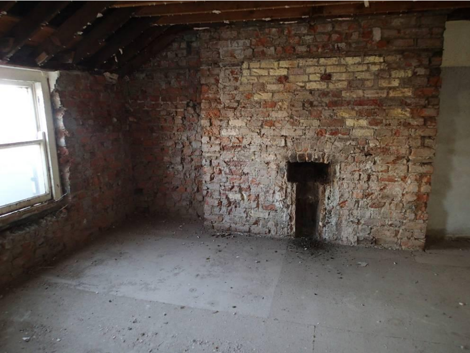
Third floor front room
