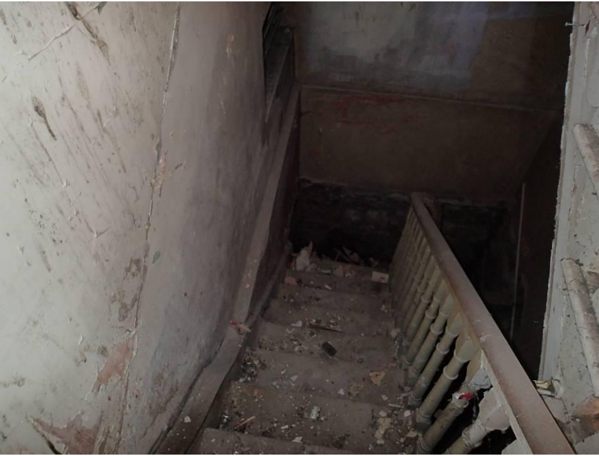
Basement staircase in return
